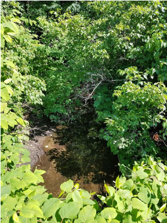
Stream channel within wetland below 6' pipe.
