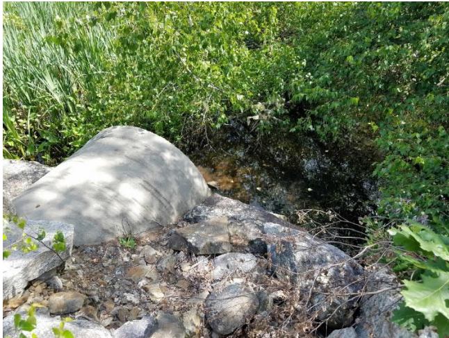
Culvert, 4' concrete, under railroad.
