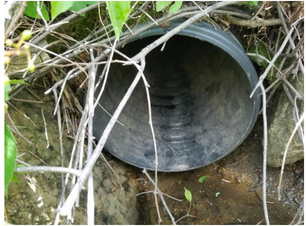
Stormwater culvert outlet at wetland
