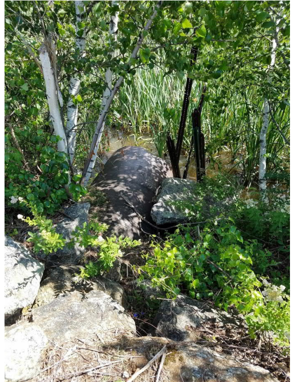
Culvert, 4', metal, under railroad.
