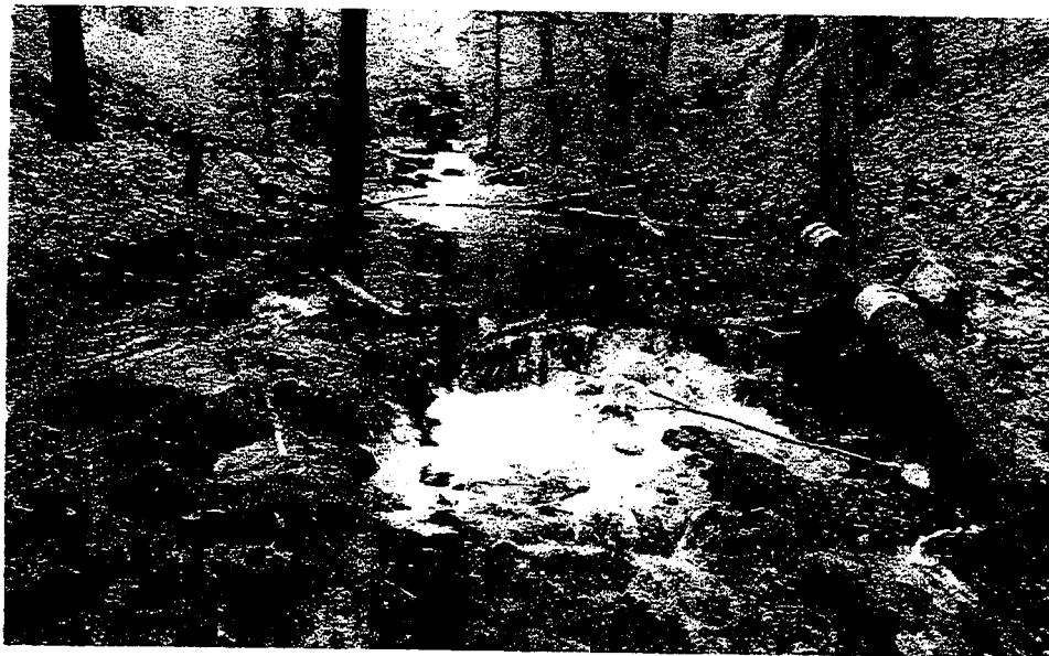
Griffin Brook, Deerfield, NH – About 3 years after installation. Added wood has created an upstream backwater, allowing the stream to reengage with it's surrounding floodplains.
