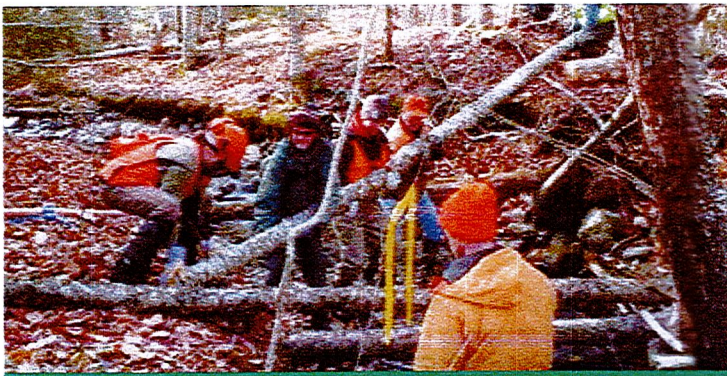
These two photos reflect the original installation and then the revisit two years later. You can see the development of the pool below the structure. This installation would involve the hand placement technique to engage the stream immediately. (Trout Unlimited photos)
